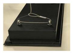
3. Feed the cable through the loop of the eye bolts. Fold the cable back forming a loop, pulling the cable through the loop on cable (see pictures).
