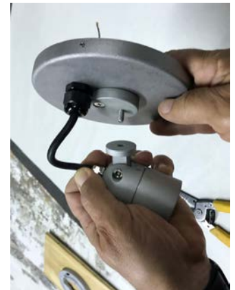
Position and screw in circular piece using screws provided and screw fixture in place (See previous page for proper alignment of screws).
