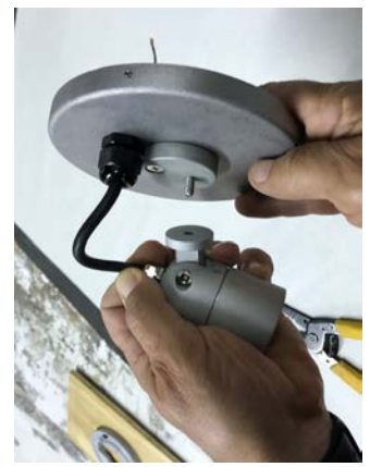
Position and screw in circular piece using screws provided and screw fixture in place (See previous page for proper alignment of screws).
