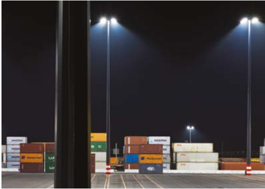
Power and efficiency - 30 lx (2.8 fc) and 45.4 kW
