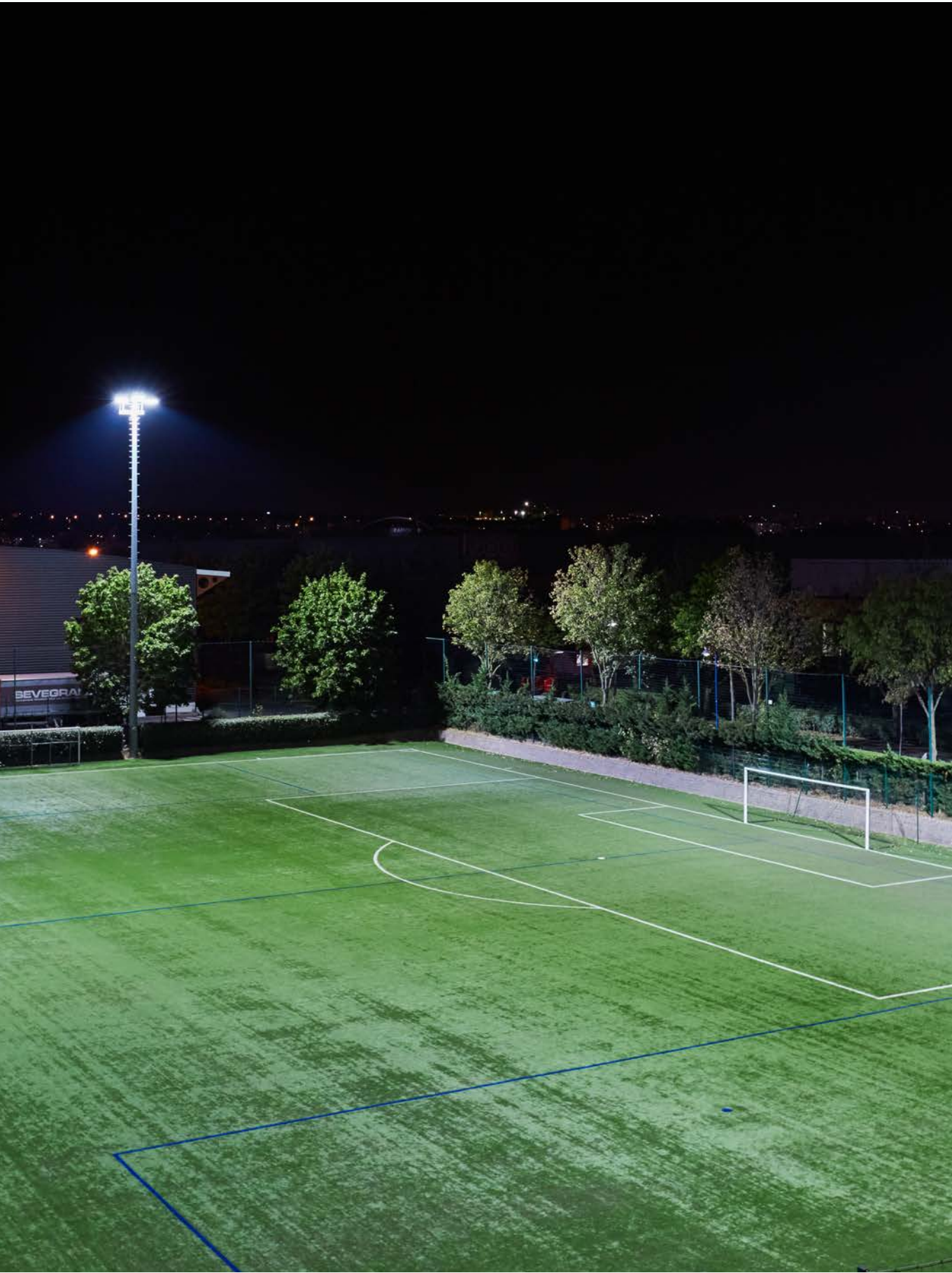
Alfortville, France / R-System gen3 MAX / Standardised according to the French National Football Association / 150 lux, U o > 0,7, E min /E max > 0,4
